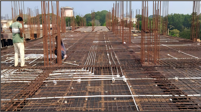
MCH - Electrical pipes in place in Second floor Slab, February, 2024.
